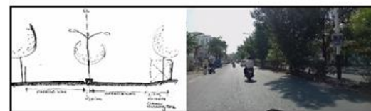
Ward - 10 Existing road section
